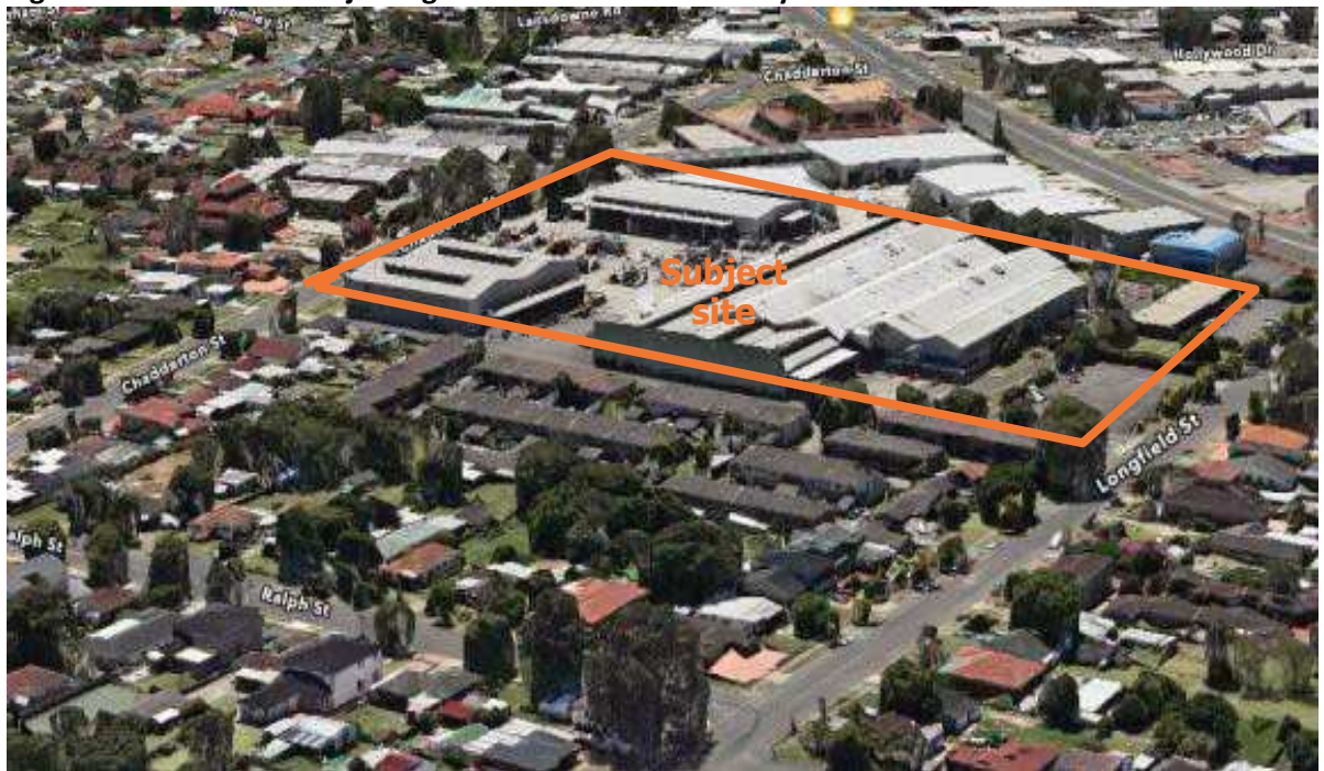
Figure 13 – Residential adjoining the western site boundary
